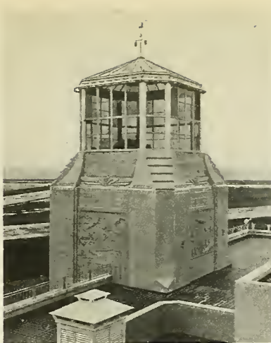
Anemometer and wind vane on control tower
